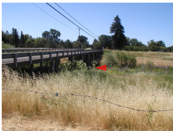
Clover Bypass from levee top, north
