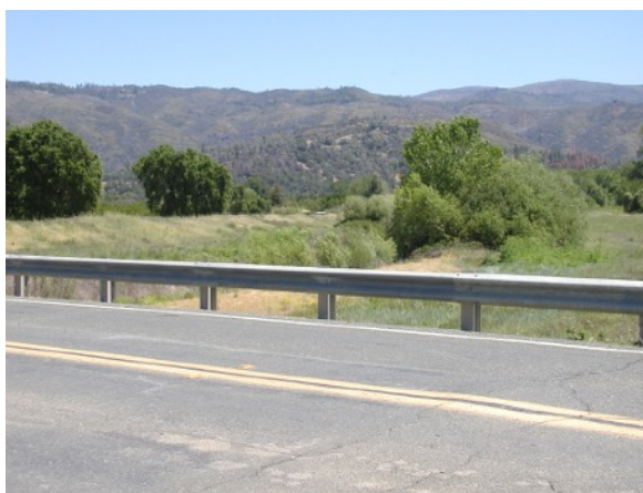
Clover Bypass upstream of bridge 5.13.21
