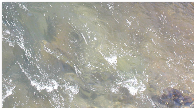
Rancheria Bridge below bridge apron, 4.18.19
